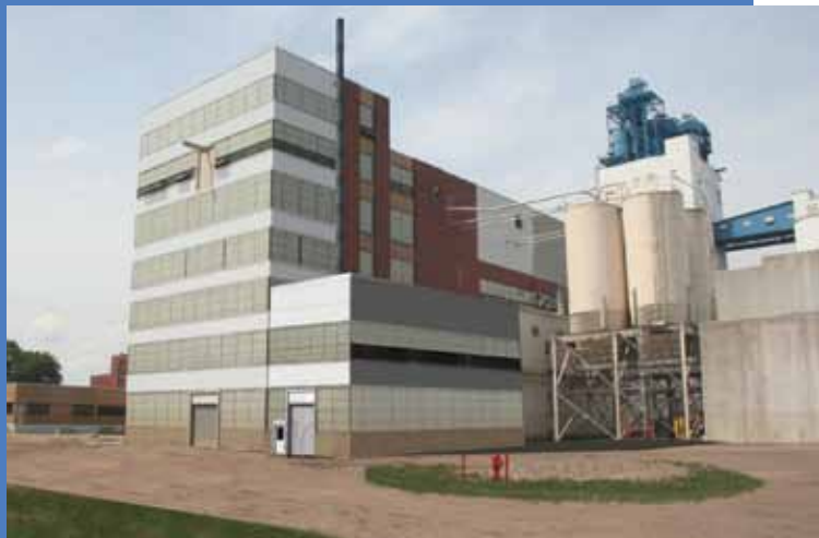
A biomass burner at General Mills' Fridley, Minn., flour mill uses 100% oat hulls to generate steam for operating the plant. Photo courtesy of General Mills
