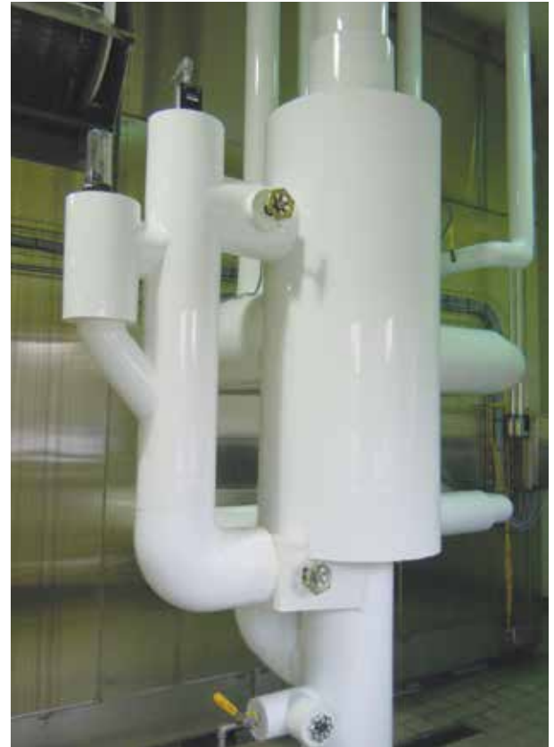
To understand the principles of refrigeration, it is necessary to have an understanding of thermodynamics. This LVS® Refrigerant Feed System from JBT Food Tech (Frigoscandia) provides liquid/vapor separation at the freezer to allow a dry suction vapor to return to the engine room, improving the compressor efficiency, reducing the system refrigerant charge, and eliminating the need for a circulation pump and surge drum. Photo courtesy of JBT Corporation
